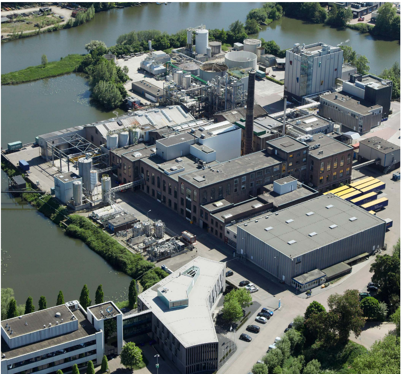
Production site at Gorinchem, The Netherlands
